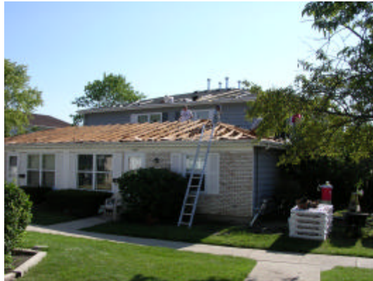
Roof decking stripped off for replacement
